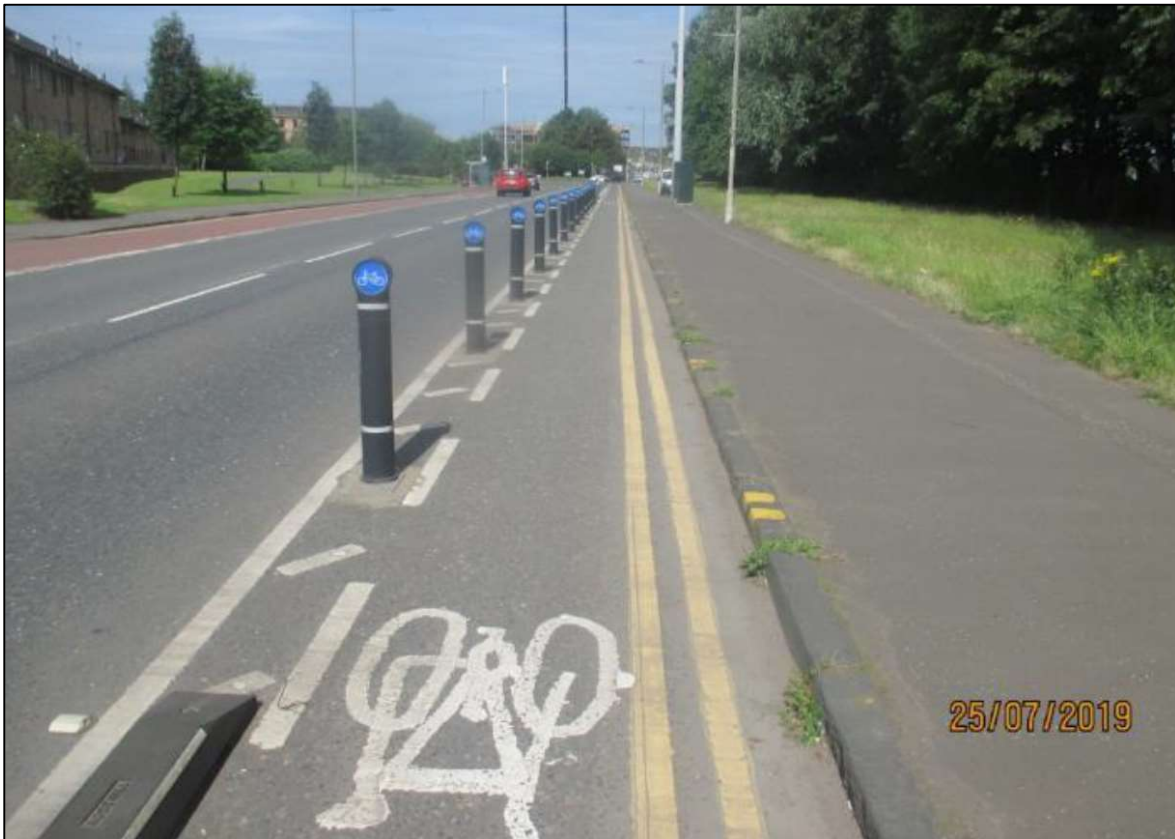
Figure 7 - Lightly segregated cycle lane/track using TSRGD 955 positioned on bollards (City of Glasgow)
