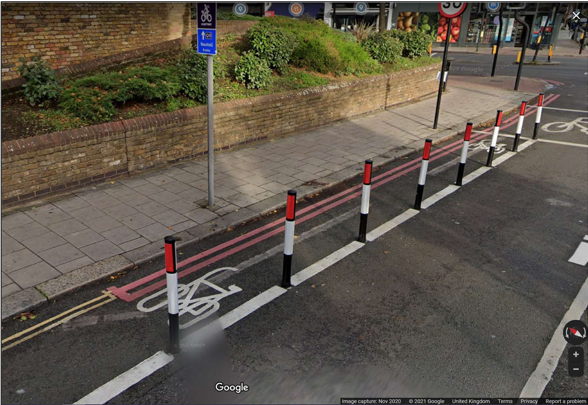
Figure 5 - TSRGD S2-6-2 sign overlapping on TLRN (Google Streetview)
