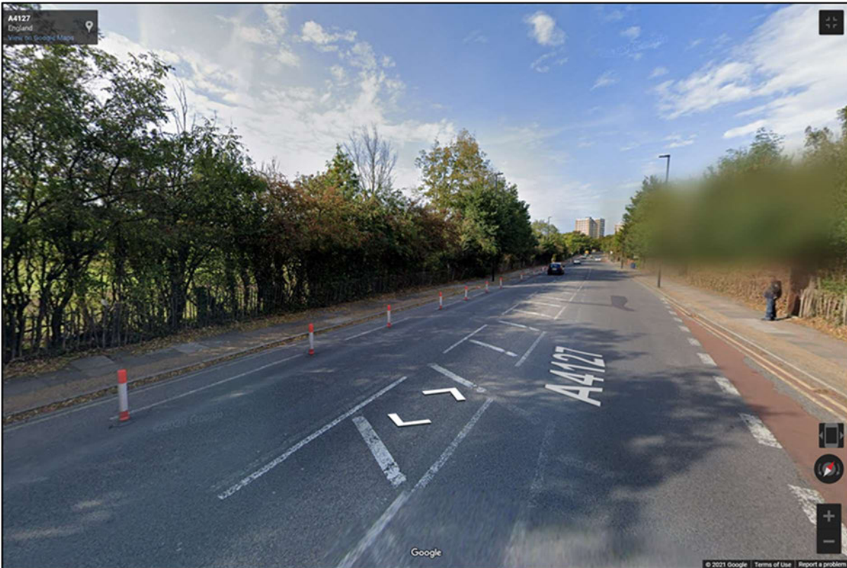
Figure 3 - Greenford Road, LB Ealing Dec 2020: use of TSRGD 7103 cylinders as a vertical light segregation feature (Google Streetview)
